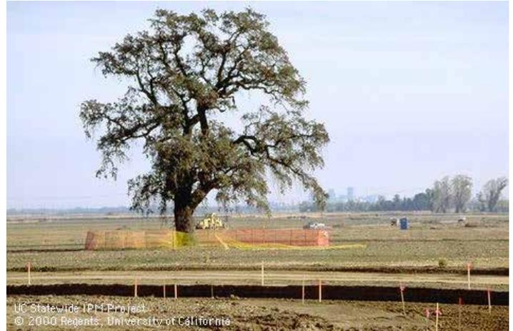
Fencing prevents damage to tree roots and trunk, and avoids compacting soil at a construction site.
